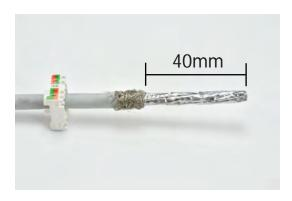
1. Insert the cable through the cap and strip the cable jacket length for about 40mm.
