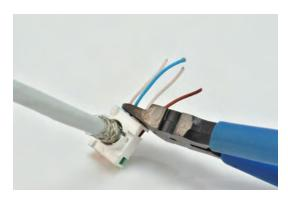
3. Trim the excess wires along the edge of the cap by using a diagonal cutter.
